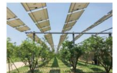
Photovoltaic Power Generation Projects Currently, We have installed 6 photovoltaic projects in Shandong and Henan, and 2 such projects are under construction
