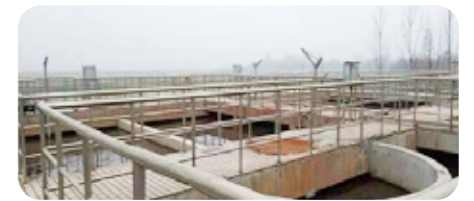
• Hydrolysis tank reconstruction scene
